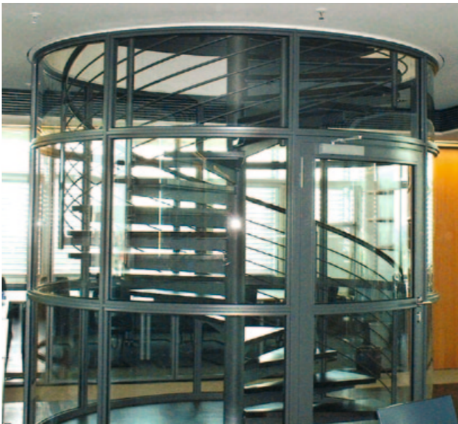
Fraunhofer Haus in Munich, PYRAN® G – Curved fire resistant glazing
