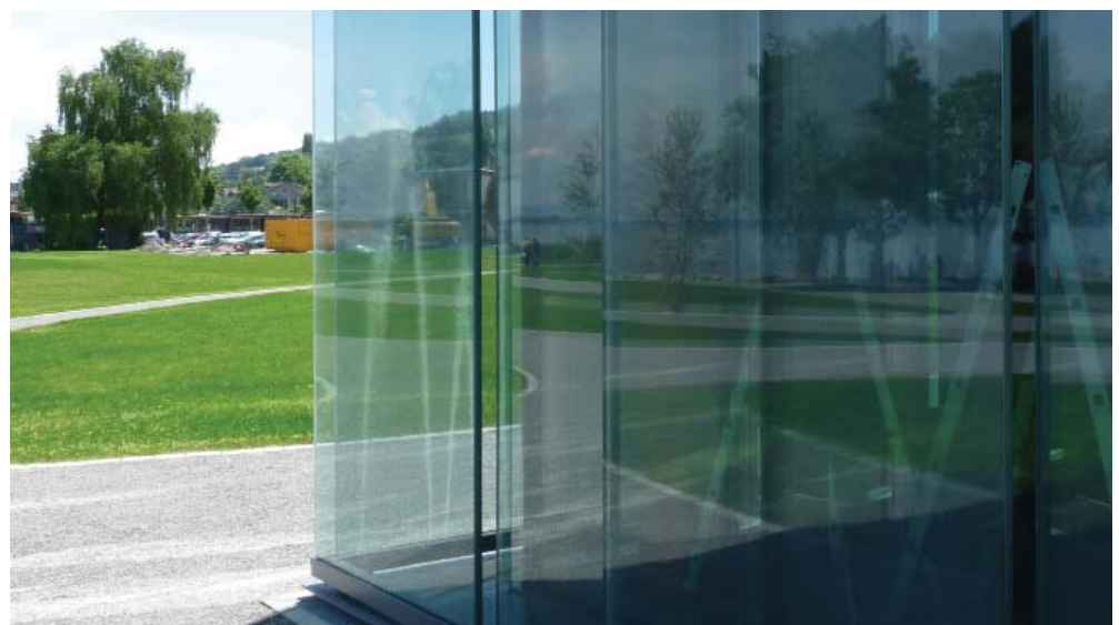
Illustration 16. Double effectivity: glazed corners become opaque and thus are much less hazardous. Birds see through transparent building corners, which is why they often attempt to fly diagonally through them.
